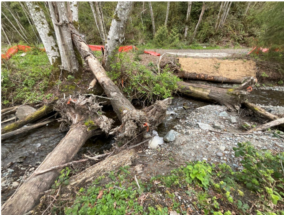
Figure 16 Large Woody Material (flagged) with Rootwads Placed in Lund's Gulch Reach 3
