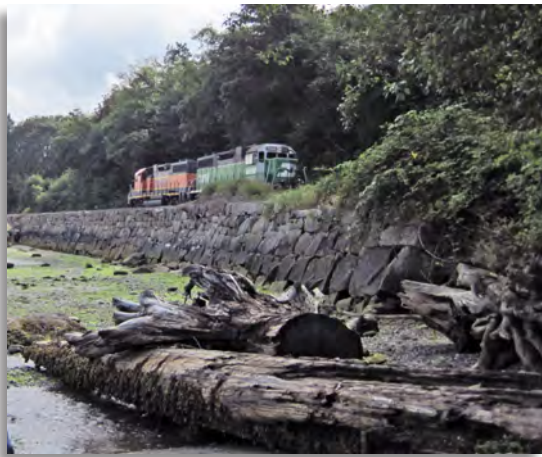
Railroad bulkhead during low tide.
